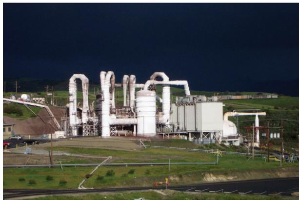
**Fig. 15** DARPA built the megawatt-class Alpha HF chemical laser during the 1980s to test prospects for an orbiting chemical laser battle station. Its ability to operate in vacuum was tested in this dedicated facility built by TRW, now part of Northrop Grumman. For scale, note the car at lower left and the sawhorse in lower center. (Courtesy of Northrop Grumman)
