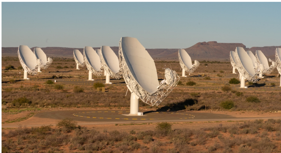
Fig. 17 Some of the 13.5-m dishes making up the MeerKAT array in the Karoo, South Africa.
