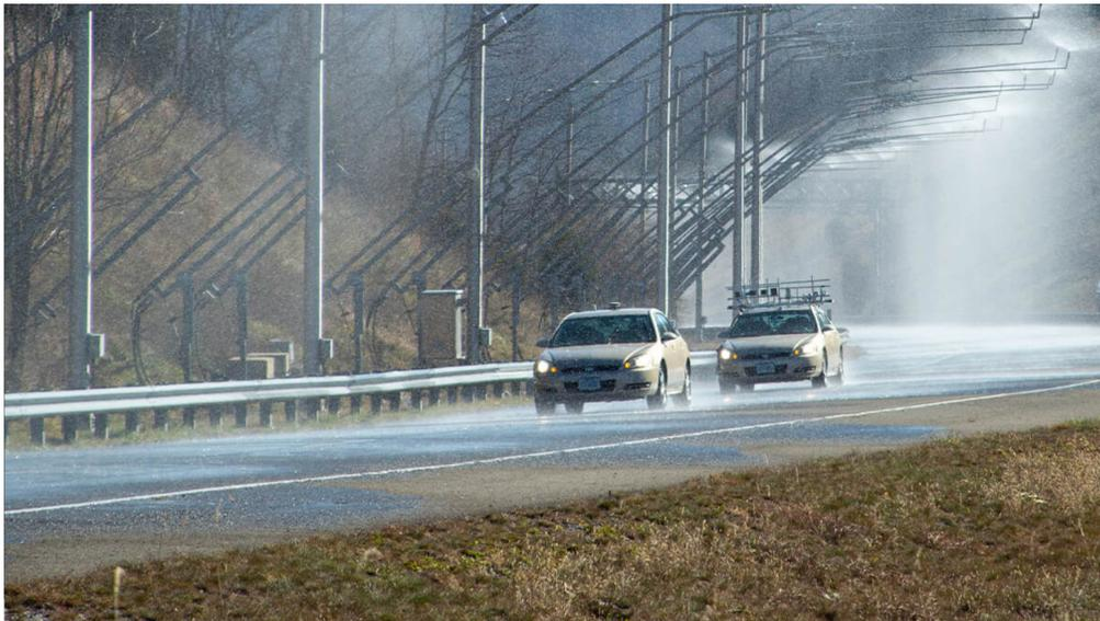
**Fig. 25** The rain testing section of Virginia Tech Transportation Institute's highway section.<sup>20</sup>
