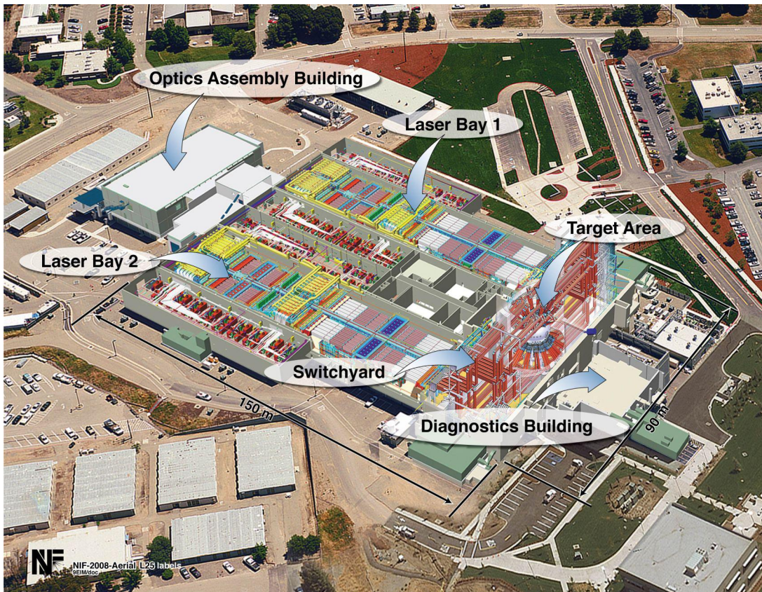
Figure 1: NIF aerial view, showing the two laser bays, switchyard, target chamber area, diagnostics building, and optical assembly building.
